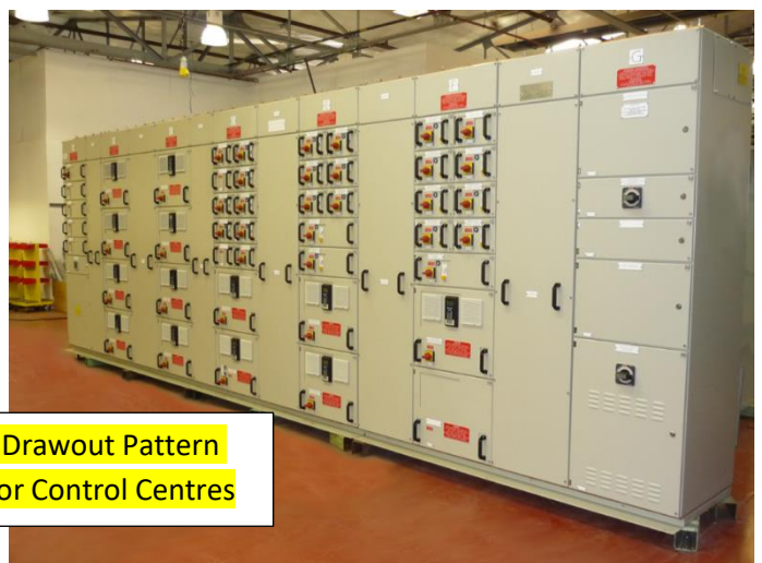
NCE Switchgear and Motor Control gear construction meets the full Seismic requirements for the UK Nuclear Industry as tested by Element Test Laboratory.
